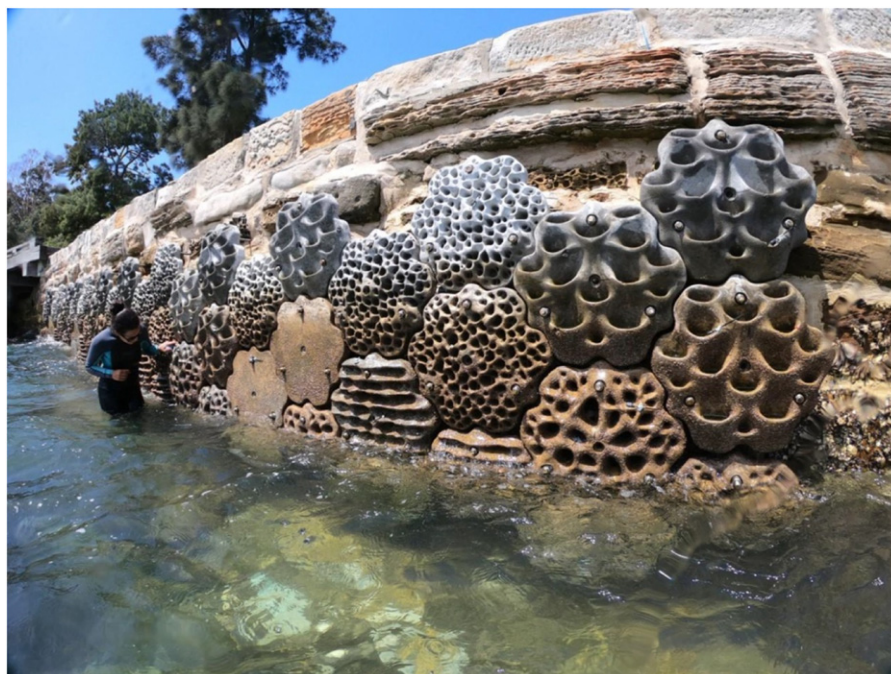
Fig. 19 A rock seawall with engineered modules installed to evaluate the responses of biodiversity to enhanced habitat complexity at different scales in Sydney Harbor Australia. Figure from Bishop, M.J., Vozzo, M.L., Mayer-Pinto, M., Dafforn, K.A., 2022 Complexity–biodiversity relationships on marine urban structures: Reintroducing habitat heterogeneity through eco-engineering. Phil. Trans. R. Soc. B 377: 20210393A.
