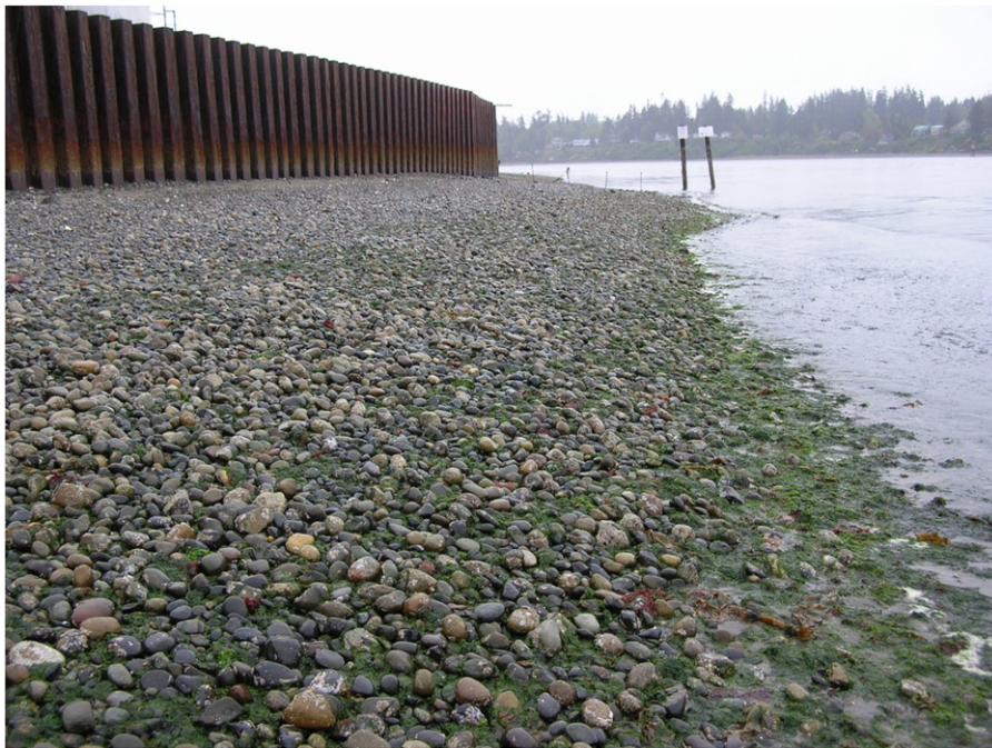
Fig. 4 An intertidal bulkhead constructed of metal sheet pilings located on Puget Sound, Washington, USA. This bulkhead was built to retain contaminated sediments and reduce exchange with the sound.
