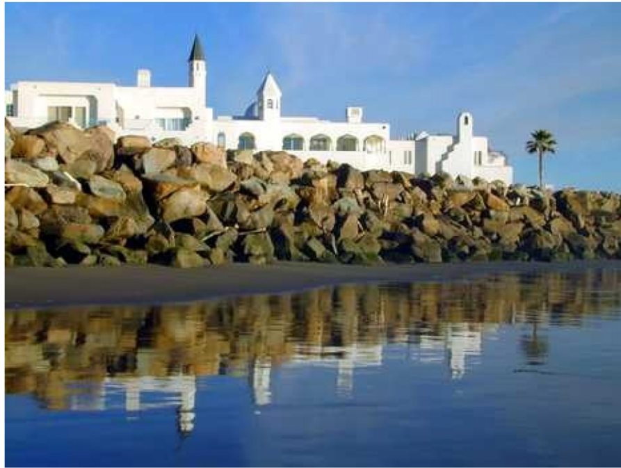
Fig. 5 An example of a rock revetment located on an open-coast beach of Santa Barbara County in southern California, USA.
