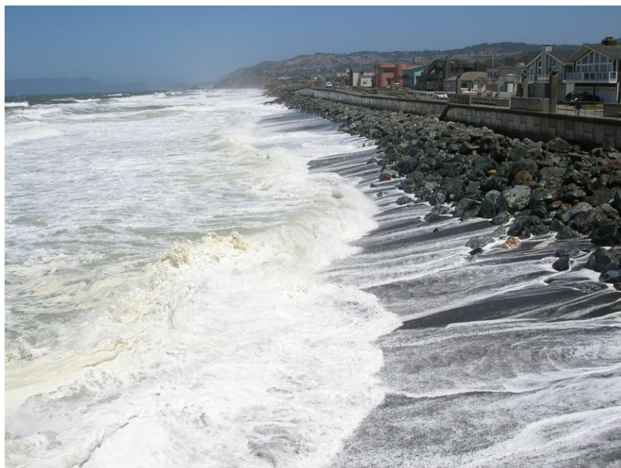
Fig. 10 Beach loss seaward of coastal armoring that includes a seawall and revetment on exposed coast in Pacifica, California, USA. Note the lack of dry sand zones and lateral access for beachgoers.
