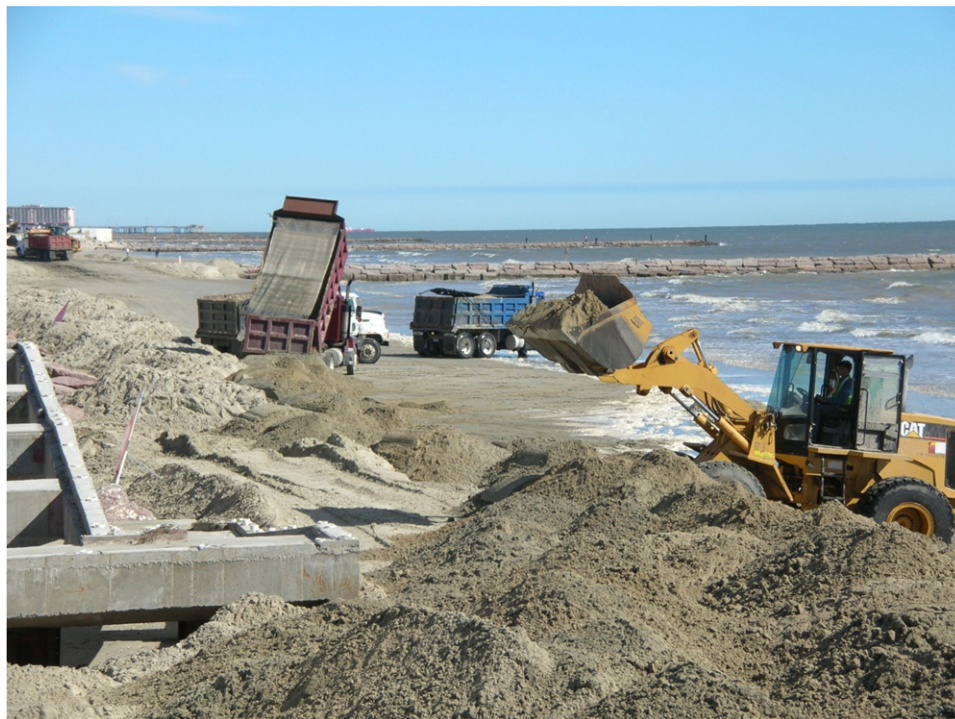
Fig. 6 Beach-filling activities between rock groynes on the open coast of Galveston, Texas, USA in January 2009 following severe erosion and damage from Hurricane Ike.
