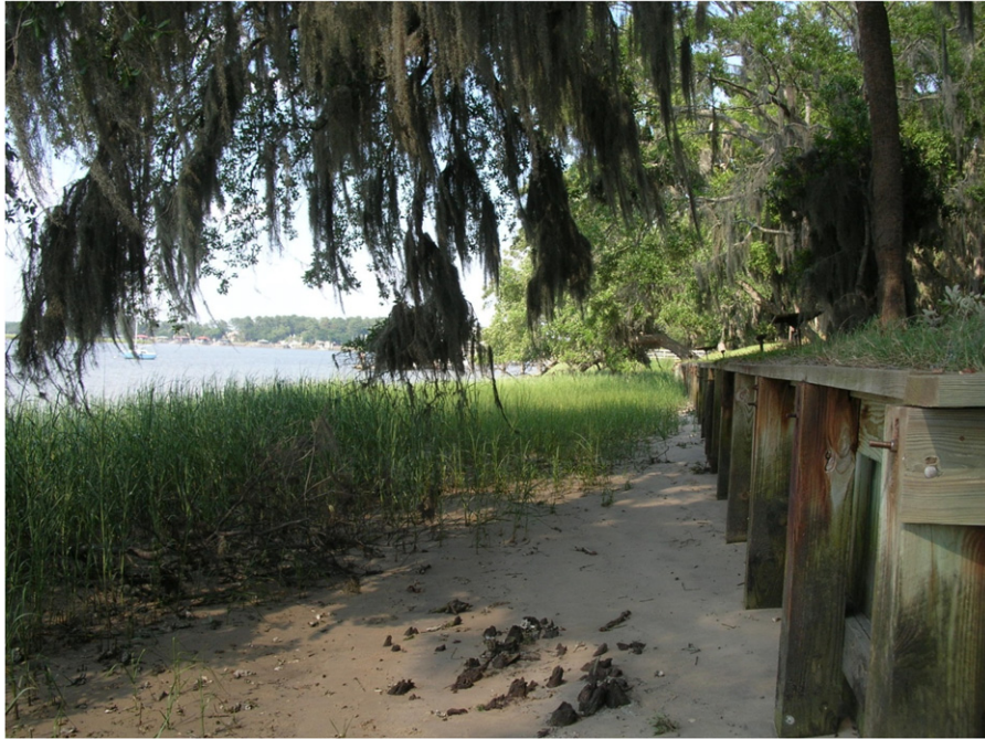
Fig. 3 A bulkhead built to protect coastal development on a sheltered shoreline, Savannah, Georgia, USA.
